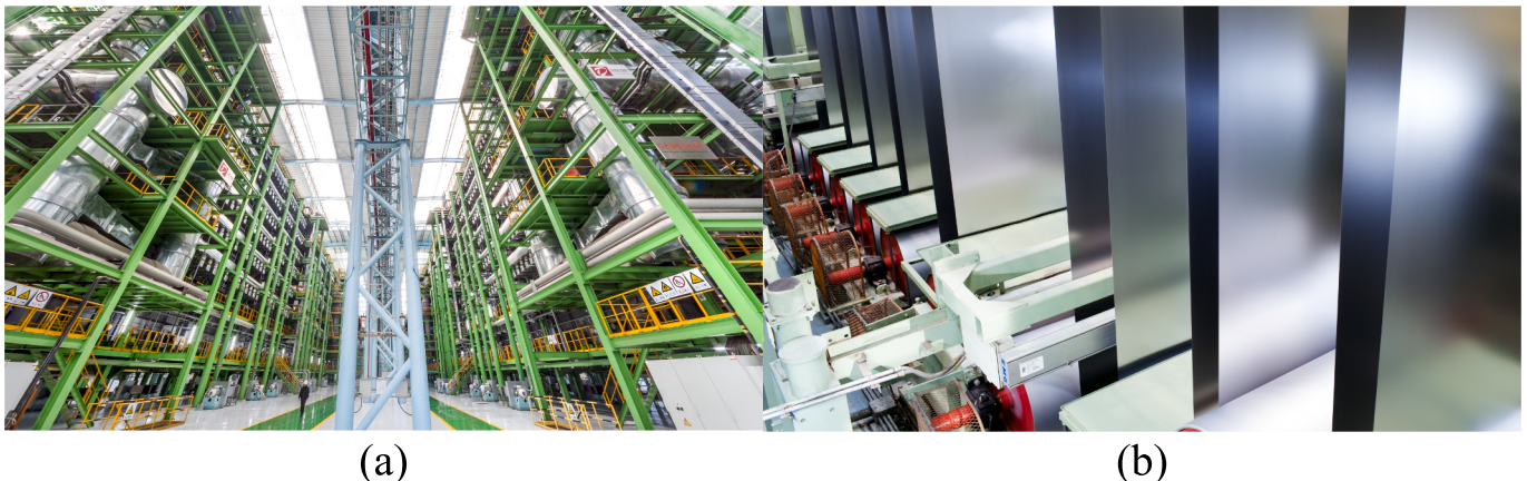
Fig. 1. Examples of continuous annealing lines for steel strip: (a) two annealing furnaces in full view and (b) detailed view of the strip accumulator [3].
