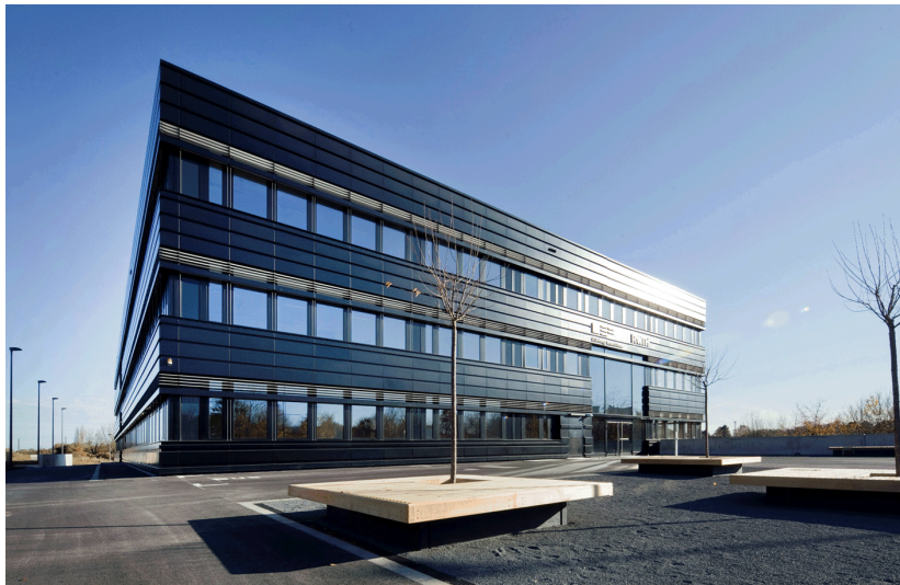
Figure 2.2: Exterior view of E.ON ERC main building
