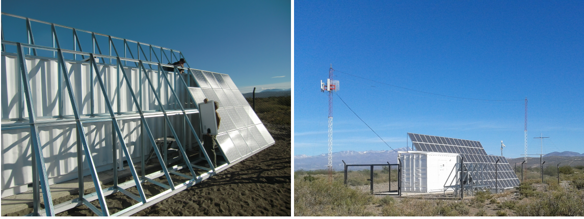
Figure 6.2: The Central Radio Station (CRS) of AERA. The left picture was taken during the installation of the solar panels which provide an autonomous power supply for the DAQ and electronics inside the sea-container. On the right photograph, the CRS in its present state is shown. The two masts and a cable spanned above the container compose a lightning protection for the CRS. The wireless communication antennas to the radio stations mounted at the left mast and a reference antenna in the background are visible.
