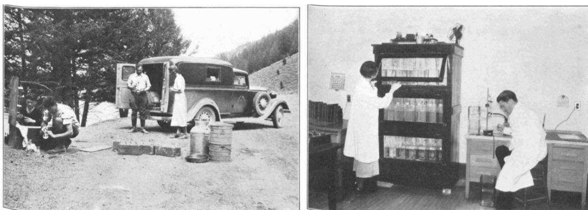
Figure 1.1: Already in the 1930s, bioassays with fish and invertebrates were applied to evaluate stream water and aquatic pollutants by the United States Bureau of Fisheries. Investigations utilized “laboratory trucks” for field work (left); and temperature-controlled cabinets for tests with Daphnia magna (right). From Ellis, 1937.
