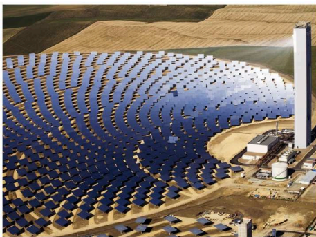
(c) Solar tower plant PS10, 11 MW in Andalucía, Spain (left), and simplified sketch of a concentrated solar tower power plant cycle using molten salt and a storage. Sources: flickr, Solar Millenium
