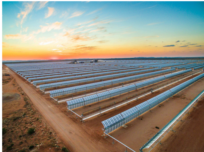
Figure 75: Network of tubes in the Noor solar power station near Ouarzazate in Morocco.
