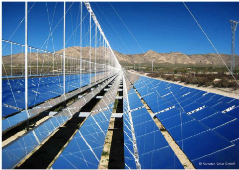
(b) Linear Fresnel collector in 1.4 MW plant PE1 in Murcia, Spain (left), and simplified sketch of a Fresnel solar thermal power plant cycle using direct steam generation (right). Sources: Novatec Solar, Solar Millenium
