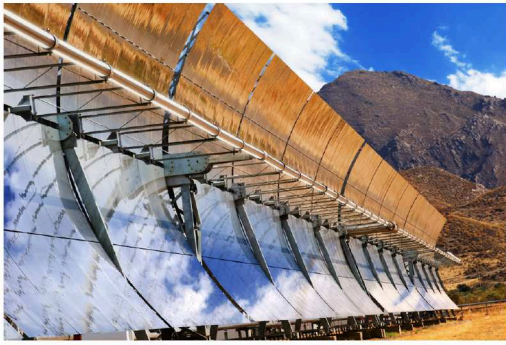
(a) Parabolic-trough solar collector at Plataforma Solar de Almería in Spain (left), and simplified sketch of a parabolic trough solar thermal power plant cycle using thermal oil as heat transfer fluid (right). Sources: DLR, Solar Millenium
