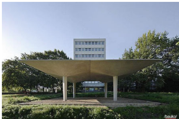
Fig. 1 Example for a textile concrete structure at the RWTH Aachen
