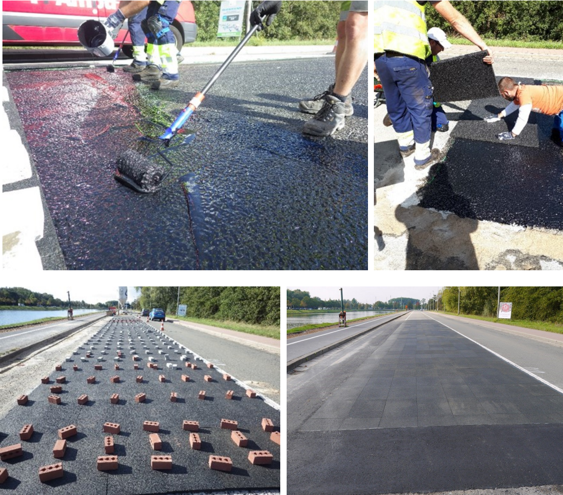
Figure 1 – The construction of the test track: spreading of the epoxy glue (upper left hand side), the placing of the slabs (upper right hand side), weights on the corners of the slabs during the drying of the glue (lower left hand side) and the finished test track (lower right hand side)
