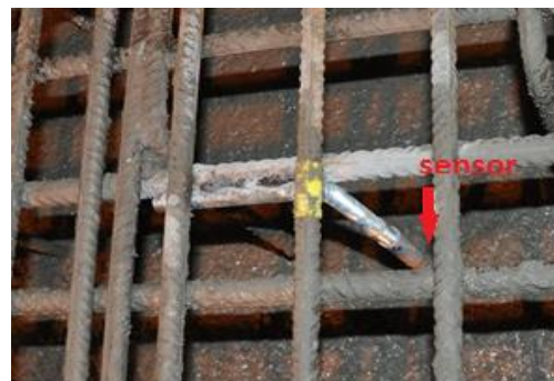
Figure 6-15: Ultrasonic transducer before concreting
