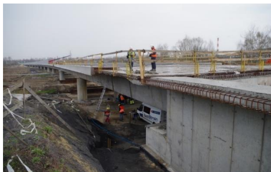
Figure 6-14: Bridge construction site in Poland.
