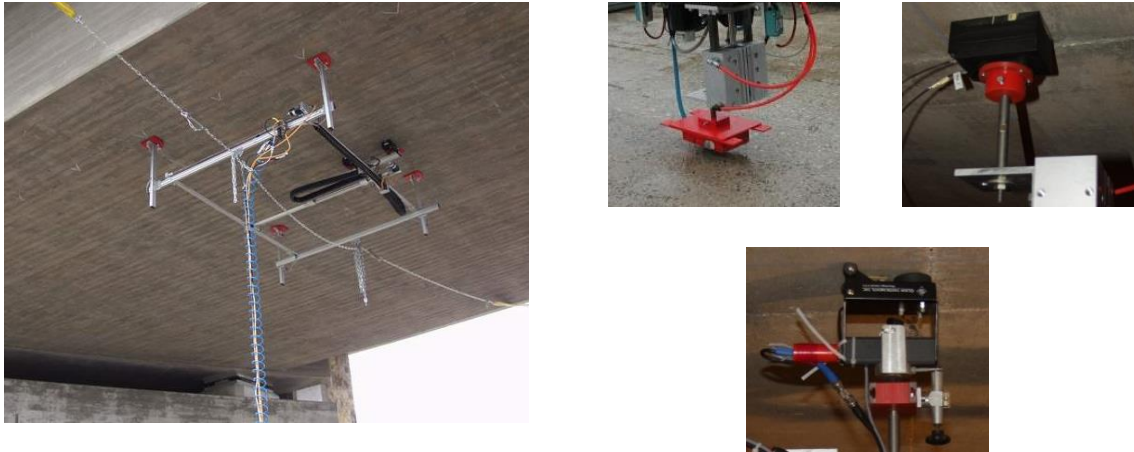
Figure 4-4: Left: BAM NDT scanning system mounted below a concrete bridge. Right: The scanners can be used with various radar, ultrasonic impact-echo or other sensors. Pictures: BAM.
