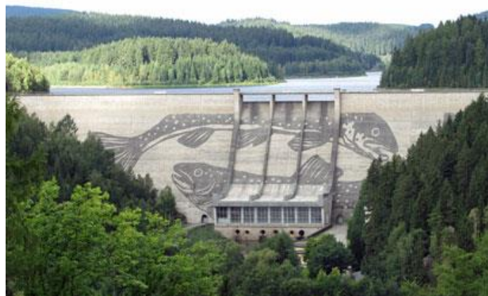
Figure 6-10: Concrete dam at Eibenstock, Saxony, Germany. Picture: Landestalsperrenverwaltung Sachsen.
