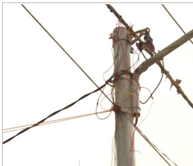
Figure 5-12 Camp residents informally splice wires from electrical poles, captured by researcher.
