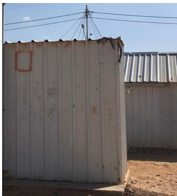
Figure 5-25 Lack of proper junctions between the walls and the roof of the caravans results in gaps from which sand and rain infiltrates, captured by researcher.
