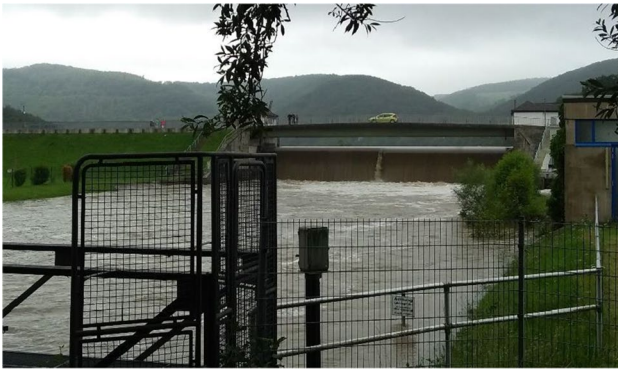
Fig. 11 Overflow over the tilting weir at the Obermaubach basin on July 15th 2021, picture was taken while collecting water samples for SSC measurements (Verena Esser, 2021)
