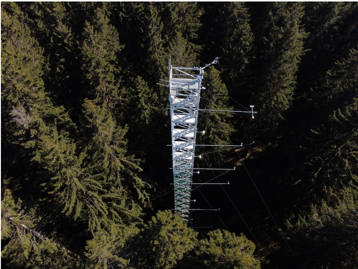
Figure 2.3 Photography of the 38 m Wüstebach tower, mounted with an eddy covariance system and sensors for photosynthetically active radiation, among others. Published with the kind permission of the authors Carsten Montzka and Jordan Bates, Forschungszentrum Jülich.
