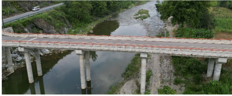
Fig. 6 Aerial view of Chi River bridge
