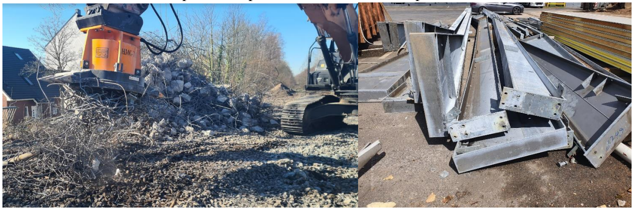
Figure 1: Steel scrap collected with a hydraulic magnet (left) and steel beams collected for recycling (right)
