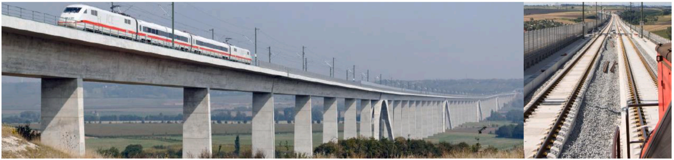
Fig. 2. Photograph of the Unstrut Viaduct.
