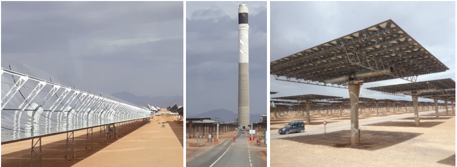
Figure 1-2: Comparative images of PTC (left), MST (center) and heliostat (right) of the Noor II and Noor III power plants in Ouarzazate, Morocco
