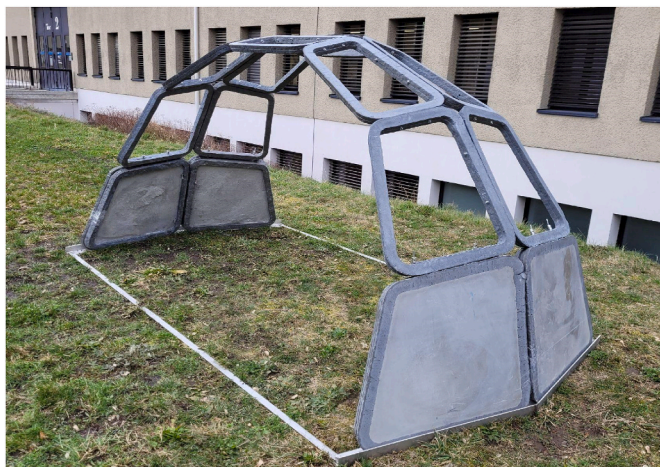
Fig. 2. Concrete shell consisting of filled and frame modules (Ivaniuk et al., 2024).
