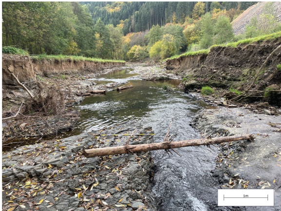
Fig. 1 Channel widening and bedrock erosion at Armuthsbach tributary 300 m upstream of its outlet, located 30 km downstream of the Ahr source. Photography shows post-flood conditions 3 months after the July 2021 event (16 Oct 2021). Post-flood channel width \approx 14 m, pre-flood channel width \approx 4 –5 m. Vertical difference between water level and floodplain \approx 1.7 m
