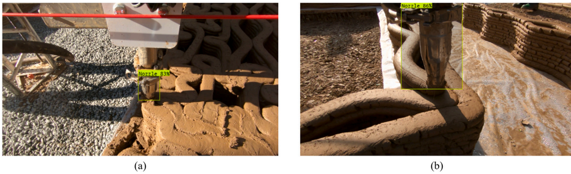
Fig. 10. Visual prediction of the nozzle from different camera angles: (a) wide-view camera, (b) near-nozzle camera.
