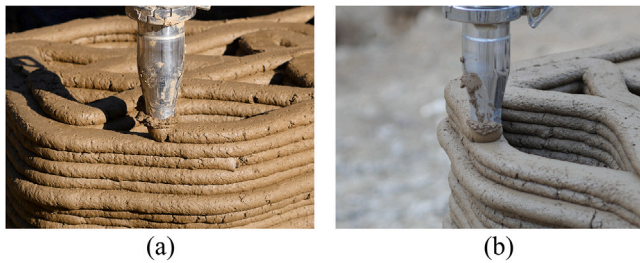
Fig. 2. Dominant lighting scenarios during on-site printing: (a) direct sunlight and (b) diffuse lighting.
