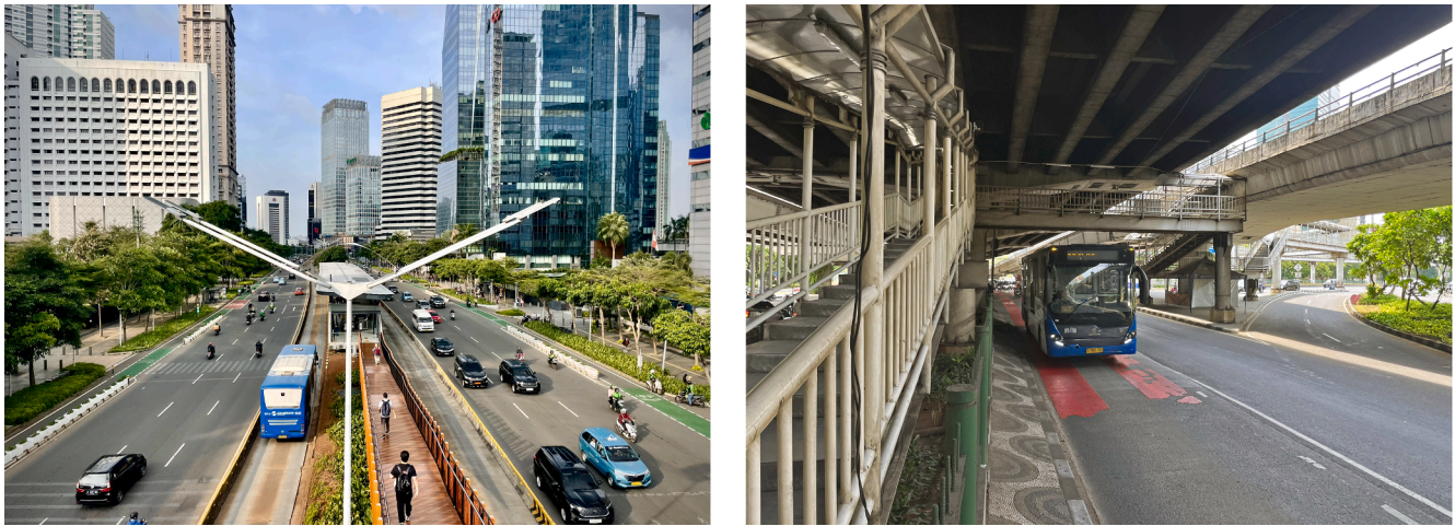
Fig. 6. Disparities in Transjakarta station design. Left: Karet Sudirman station (Corridor 1, South Jakarta). Right: Simpang Cempaka station (Corridor 10, North Jakarta). Photos: Franco Jauregui-Fung (2024).
