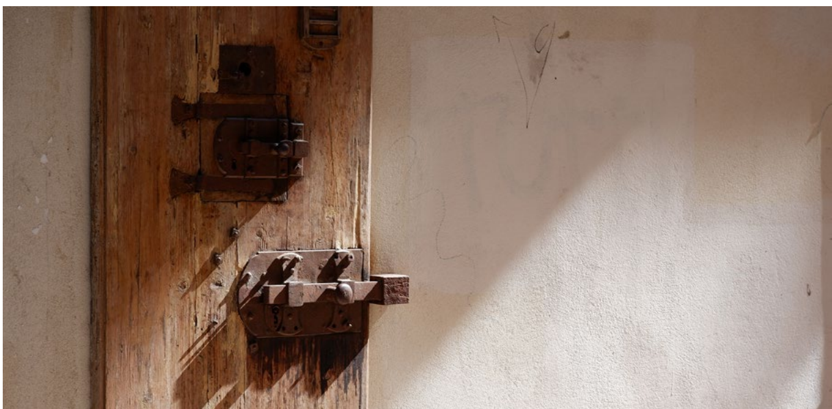
Figure 5: Original wooden cell doors. Photo: Constanze Wolfgring.
