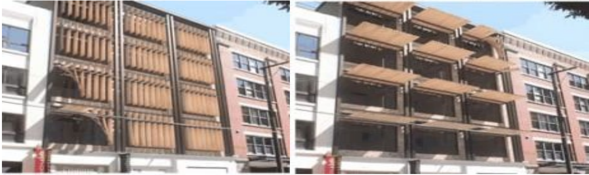
Figure 1: Kinetic façades move in three dimensions to screen sunlight from any angle [8]
