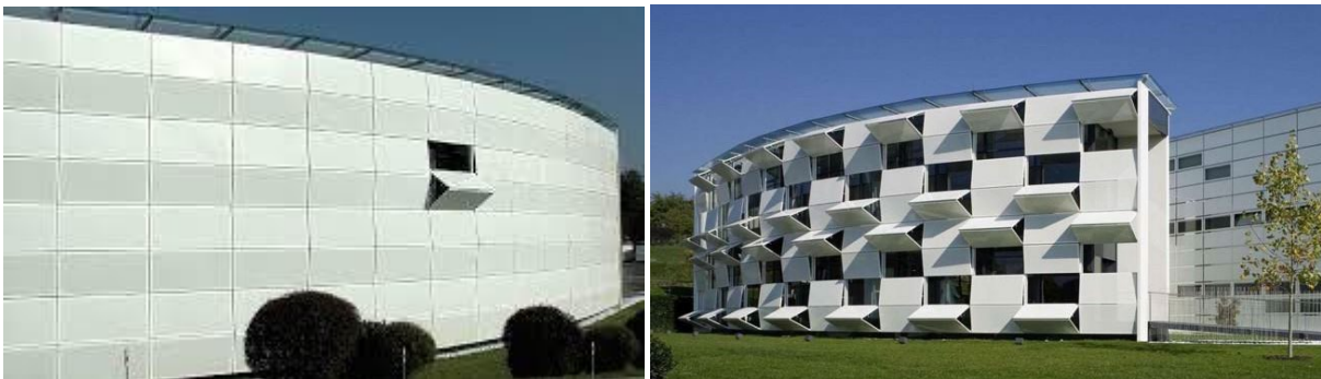
Figure 2: The Kiefer Technic Showroom in Bad Gleichenberg [9]
