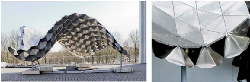
Figure 6.1.: Left: Hexagon-based point-folded structure of the freeform TRADEFAIR design. Right: Close-up of hexagon-based pyramids connected by triangle panels. Images courtesy of the Chair for Structures and Structural Design ( http://trako.arch.rwth-aachen.de ) and the Institute of Metal Forming ( http://www.ibf.rwth-aachen.de ).
