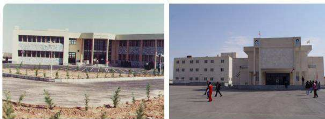
Figure 3.3 Girl high school (left) and new technical school (right) in Sangam town
