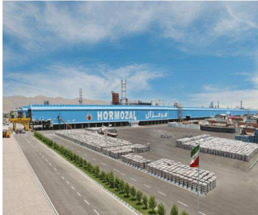
Hormozal Aluminum Plant
