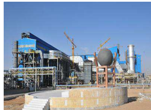
Gol-e-Gohar Pelletizing Plant
