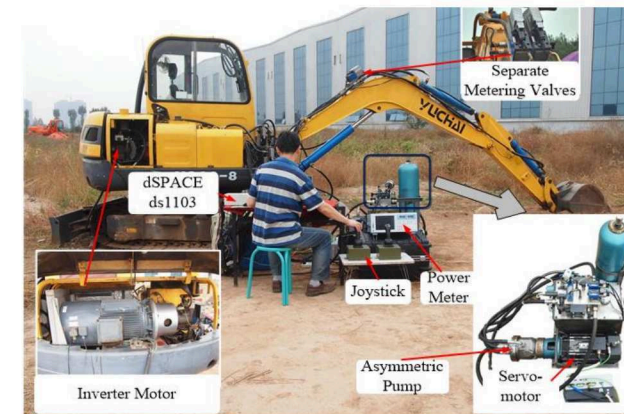
Fig.5 Photograph of mini-excavator with the proposed system
