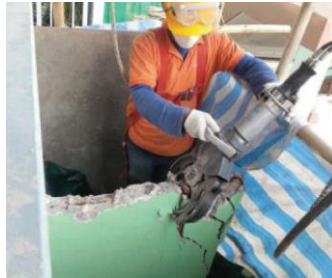
Figure 13 – Hand-held concrete crushers can be used for concrete breaker
