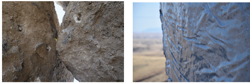
Figure 16 – Structures of Landscape , Left: Porous concrete surface finish, Right: Smooth concrete surface finish
