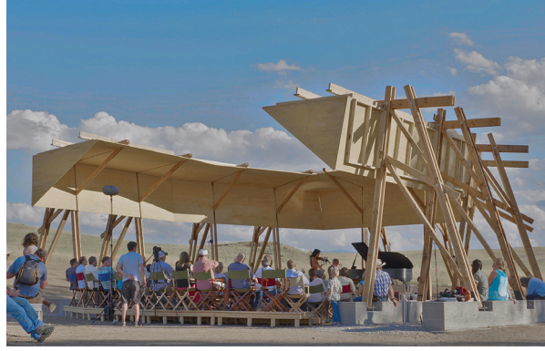
Figure 2 – Tiara Acoustical Shell ©2
