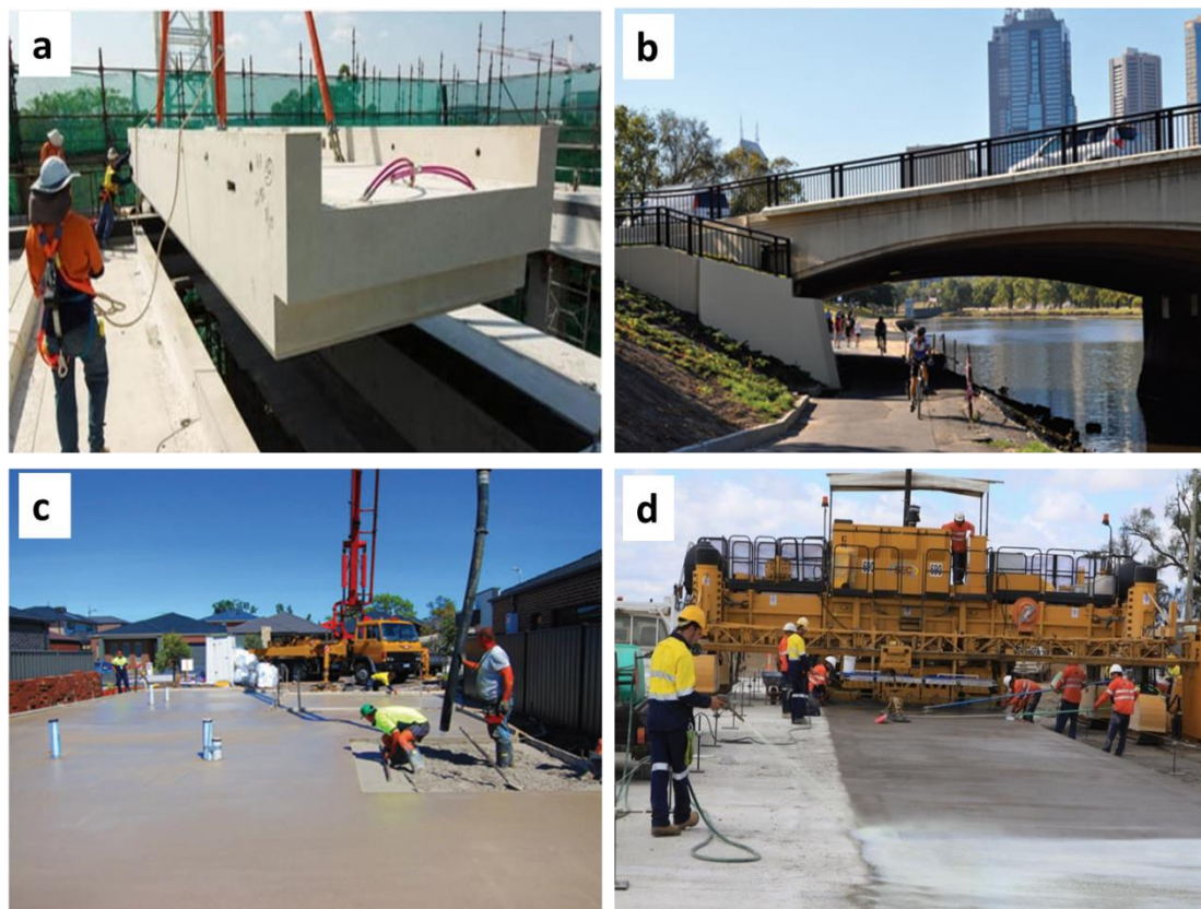
Fig. 5 Application examples of geopolymer concrete: (a) precast panels [37], (b) retaining wall surrounding a bridge [1], (c) residential housing slab [1], (d) in-situ cast aircraft pavement [38]
