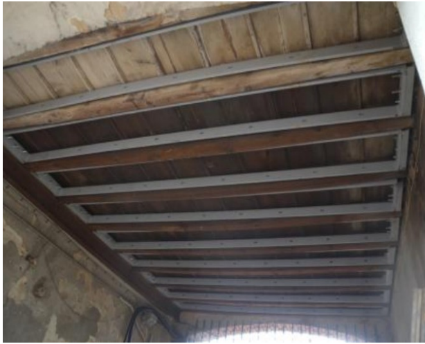
Fig. 6-8 (left) Wooden roof is reinforced with steel to maintain the original structure. Photographed by the author in 2018.
