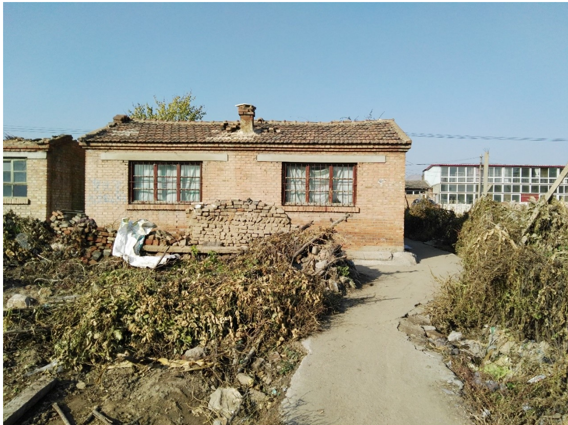
Fig. 3-7 Typical single-storey building in the study area.
