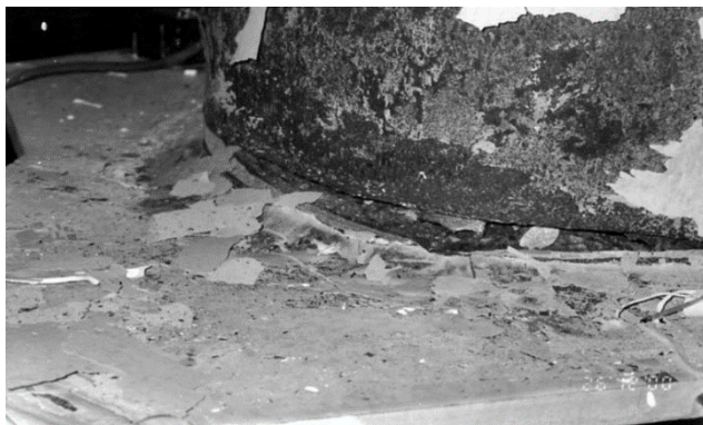
Figure 2.4 Welding fracture at column welds (Cheng and Chung 2003)
