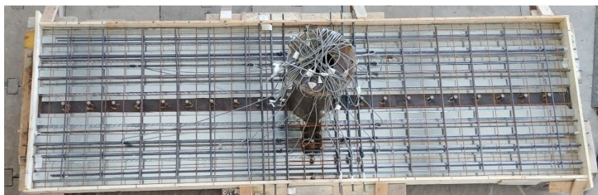
Figure 7.30 Formworks of a four-way specimen
