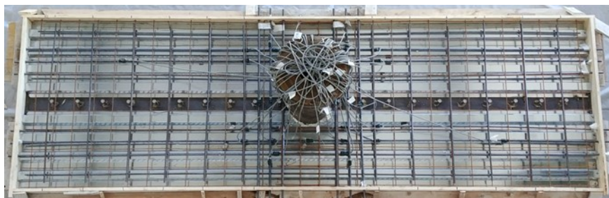
Figure 7.29 Formworks of a two-way specimen
