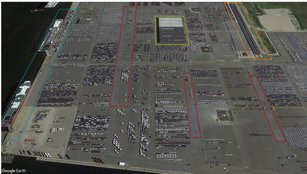
Figure 2.2: Example showing a compound with a rail track, a vessel quay and a VMC. Vehicles are stored in lanes or a fish-bone pattern and moved around for loading / unloading and services (Source: satellite image from Google Earth 2021).
