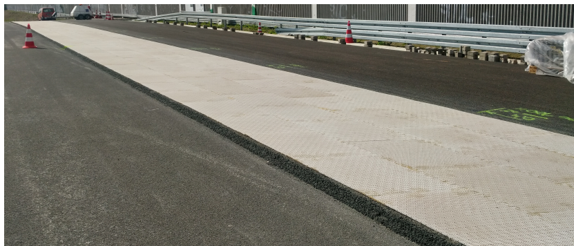
Figure 5.9: Full-scale two-layer pavement system after construction.
