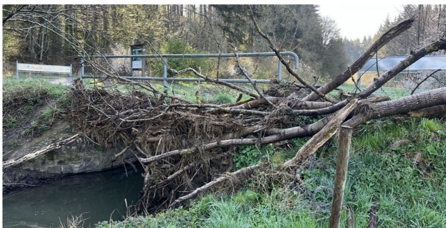
FIGURE 2 Exemplary photo of a bridge in the upper reaches that showed indication of clogging during the flood event (own figure).
