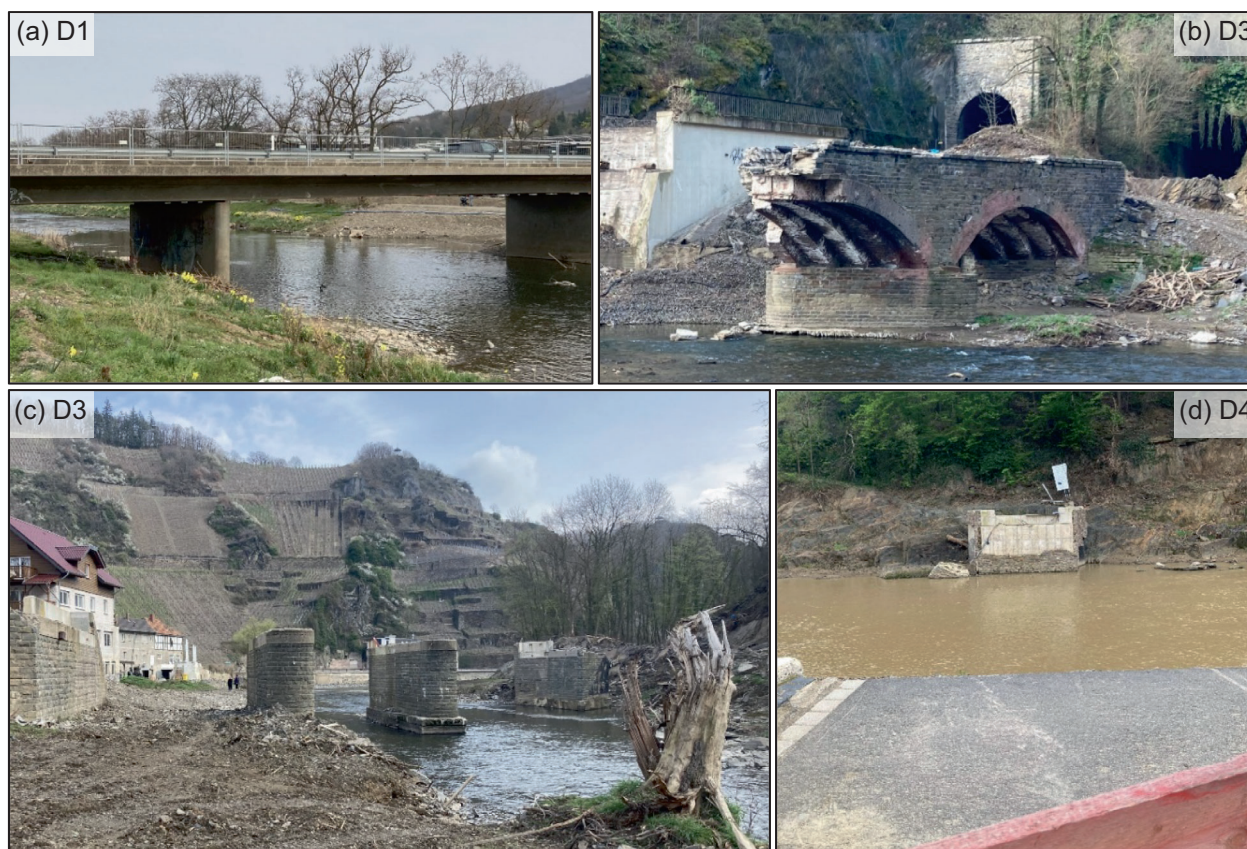
FIGURE 6 Documentation of different damage classes along the river Ahr: (a) loss of handrail, (b) large scale removal of building fabric, (c) loss of the superstructure, and (d) complete collapse (own figures).
