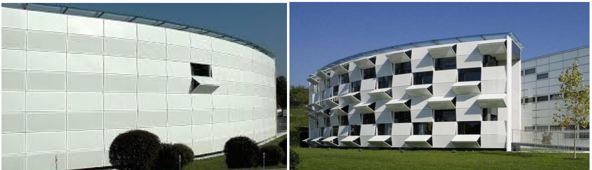
Figure 2: The Kiefer Technic Showroom in Bad Gleichenberg [9]
